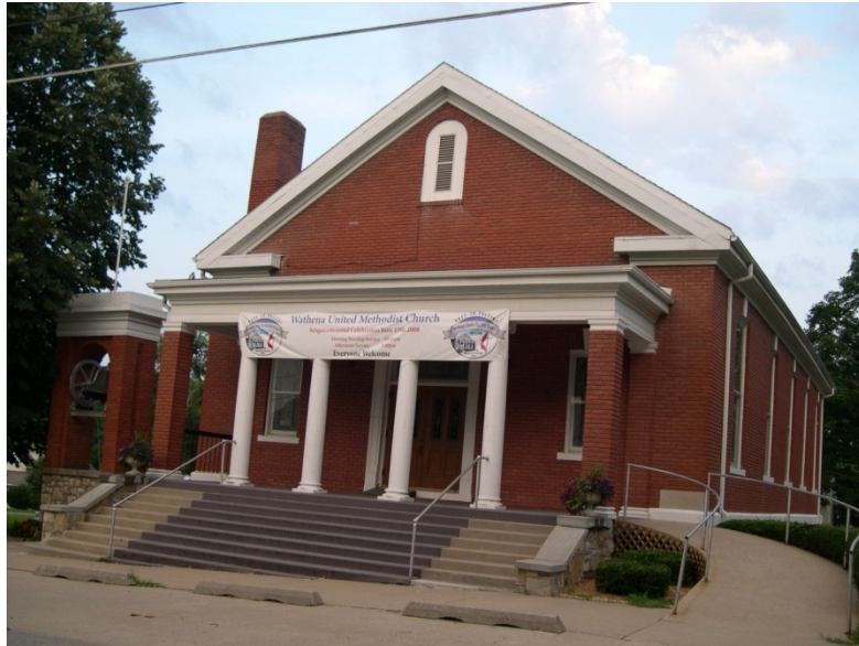
Picture of current Wathena United Methodist Church Building Courtesy of the Wathena United Methodist Church Archives
